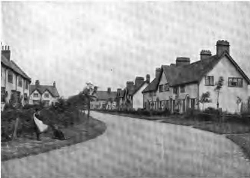
Illus. 226.—Poplar Grove, Earswick, showing a simple and economical treatment of road. Published by courtesy of Mr. F. W. Sutcliffe, Whitby.
