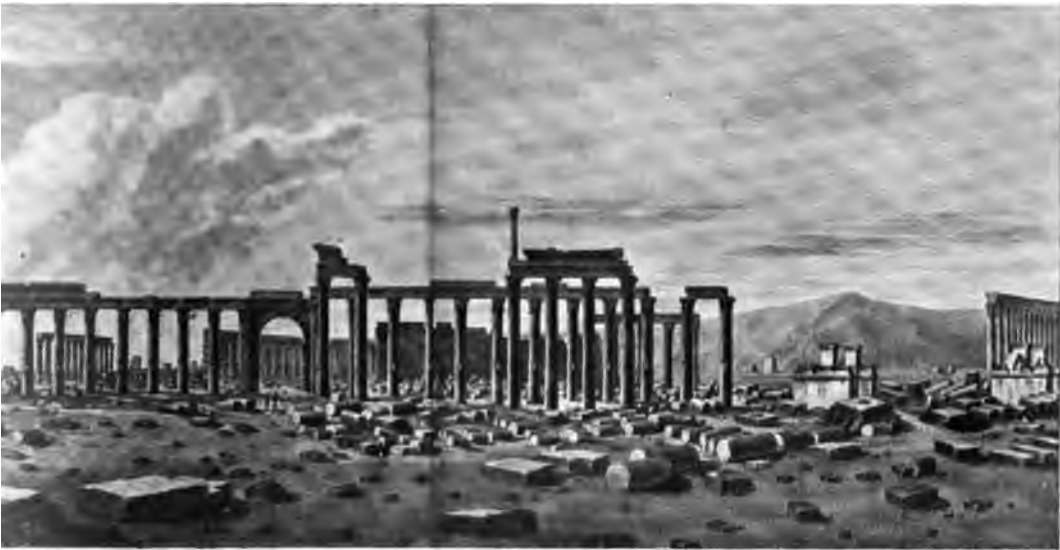
from the building marked "C" on the left of the plan to the pedestals marked "D."
