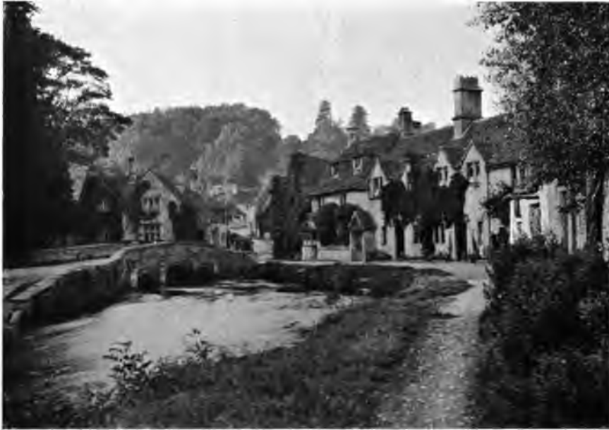
Illus. 86.—View showing informal development.
