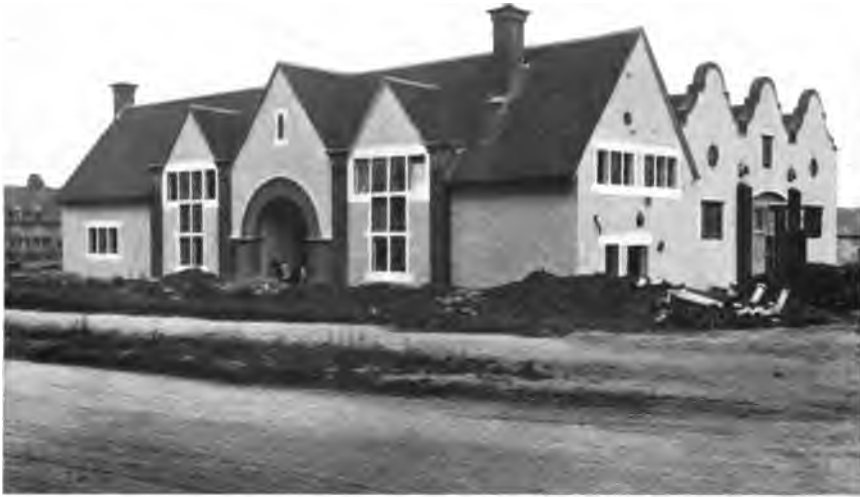
Illus. 103a.—The St. Edmundsbury Weaving Works, Letchworth. Barry Parker and Raymond Unwin, Architects.
