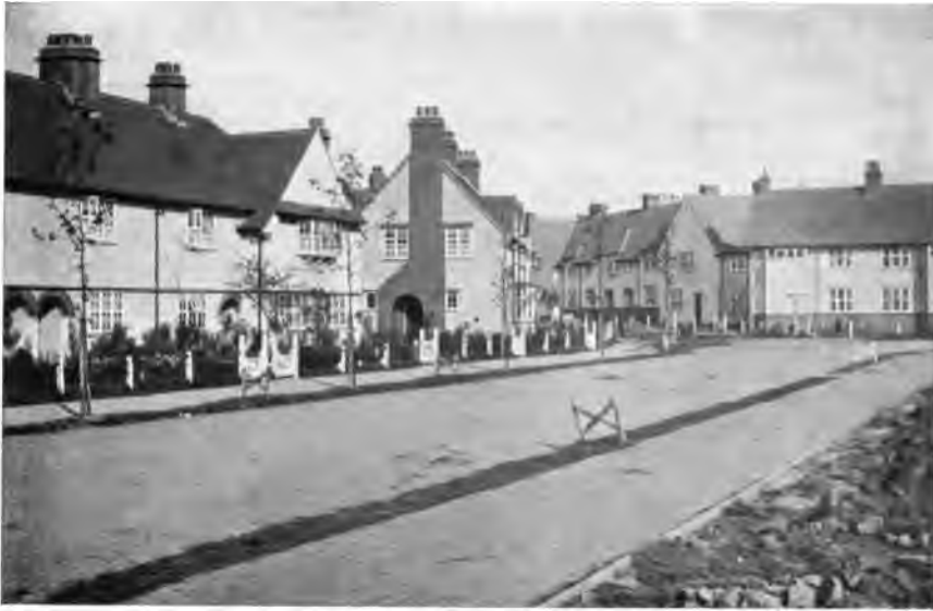
Illus. 257.—Hampstead Garden Suburb. Photo showing road junction treated as plan Illus. 253. Photo taken by Mr. J. P. Steel, Stoke-upon-Trent.
