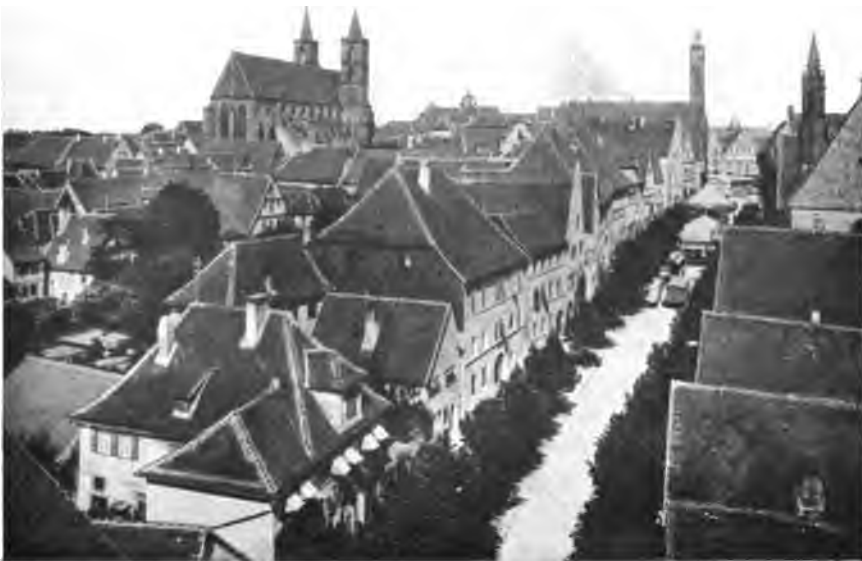
Illus. 285.—Kothenburg. Standpoint X on Fold Plan III., view showing general harmony of buildings.
