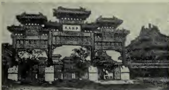
Memorial arches, such as this in the Summer Palace, are put up by special authority to commemorate the great. They are generally built of wood.
