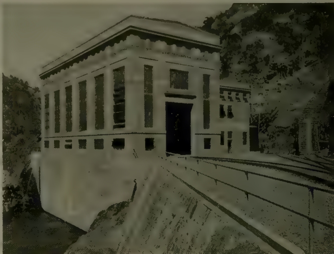
Melones Power House, on the Stanislaus River below Melones Reservoir.
