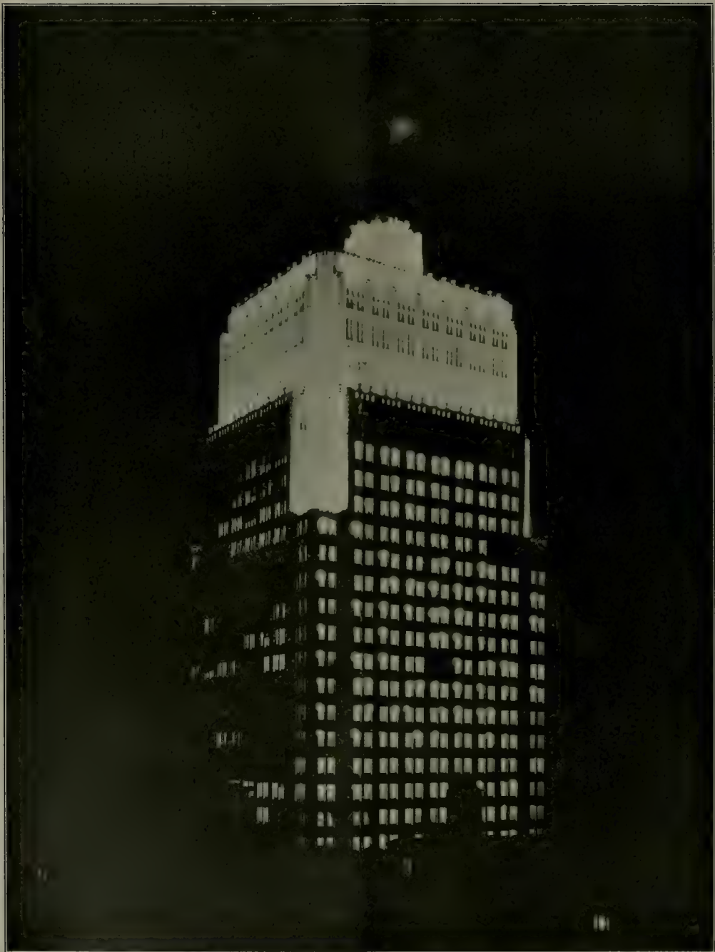
Telephone Building 140 New Montgomery Street
