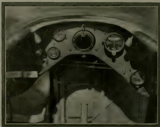
Instrument board, Boeing Air Transport Transcontinental Mail Plane.
