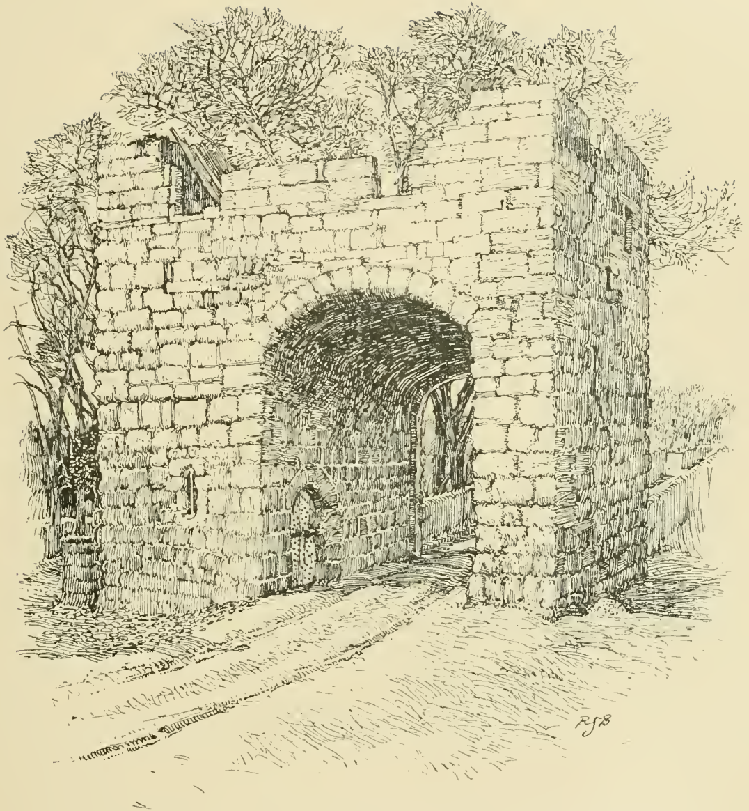
GATEWAY AT SOUTH END OF WARKWORTH BRIDGE.
